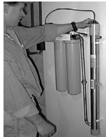
Install UV unit
